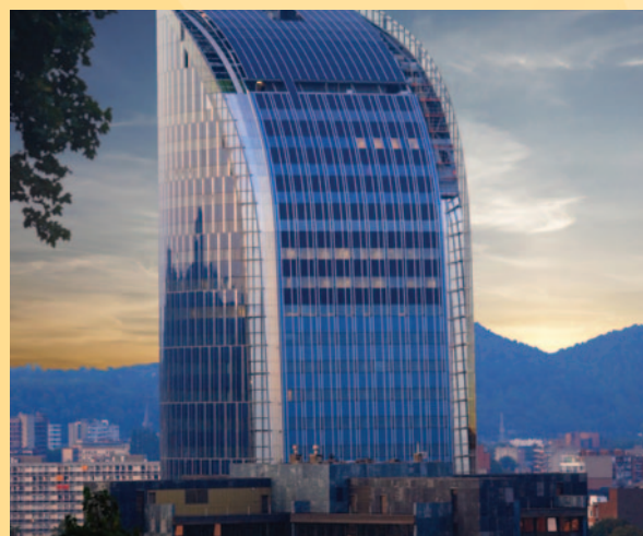
FINANCE TOWER, LIÈGE, BELGIUM, BIPV BY ISSOL, SIMCO ITALIA, JASPERS EYERS ARCHITECTS
